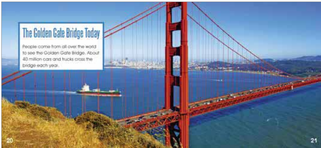
Sample taken from Golden Gate Bridge
